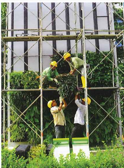
Installation of VGM®
