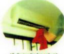
12. Drying the fan coil unit
