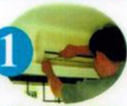
1. Dismantling of fan coil cover
